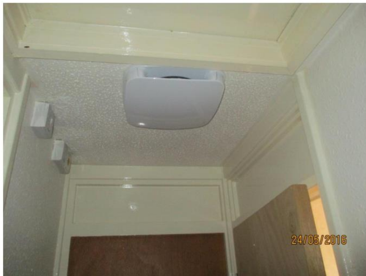
Fig. 6 – Recently installed positive pressure ventilation unit to landing.
