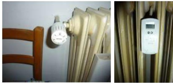
Figure 29 Thermal expansion valve and meter in a radiator
