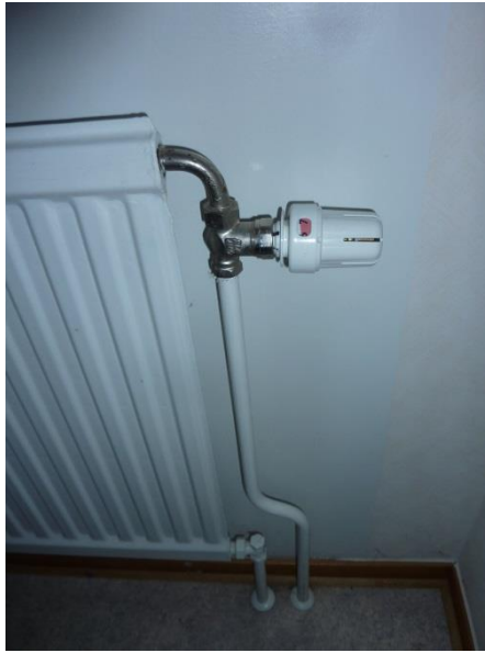
Figure 102 Regulation in a radiator
