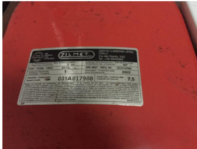
Figure 64 Expansion vessel
