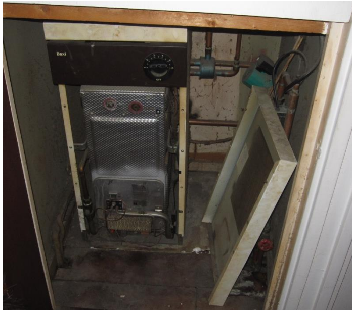
Figure 19 Gas boiler
