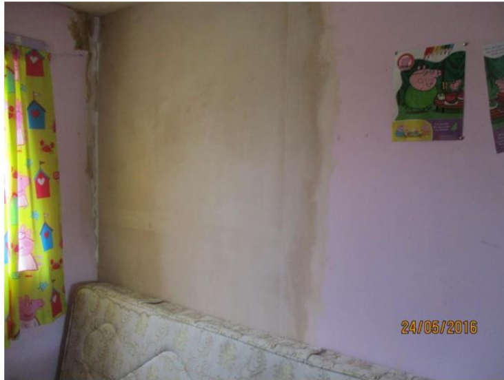
Fig. 5 – Re-plastered wall finishes to Bedroom 2.
