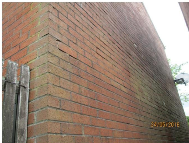
Fig. 2 – Gable elevation with defective pointing to brick work.
