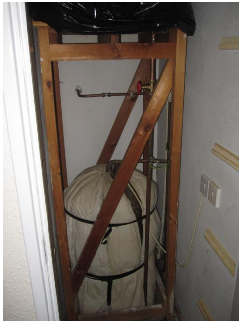
Figure 17 Electric boiler
