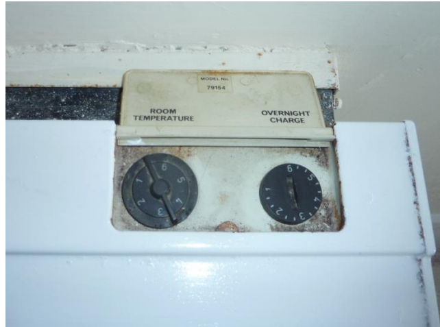
Figure 23 Regulation of the night storage unit
