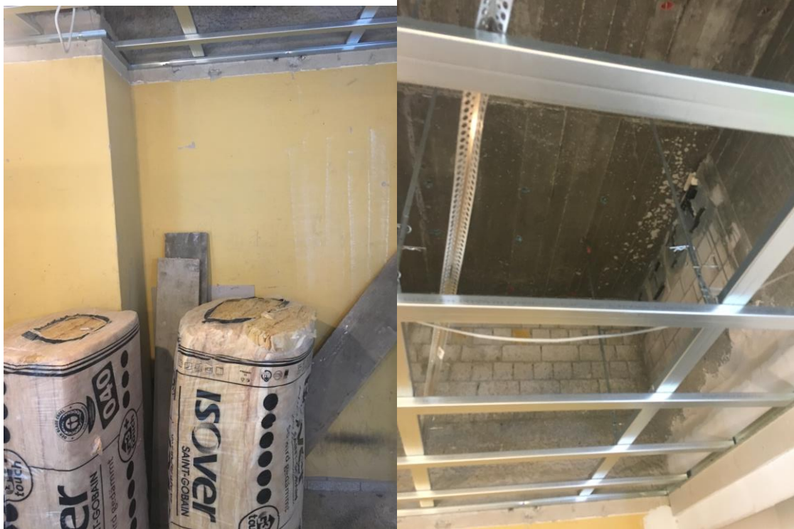
Figure 13. Ground floor ceiling insulation being applied
