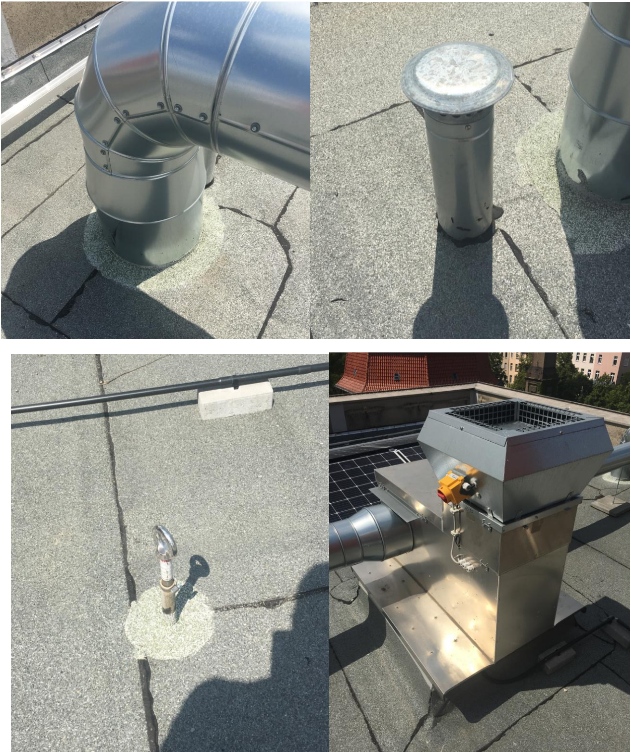
Figure 4. Sealings around perforations in the roof envelope
