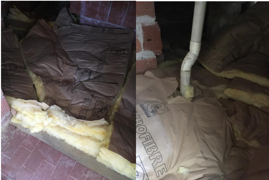
Figure 36. Cold attic insulation with mineral wool mattresses
