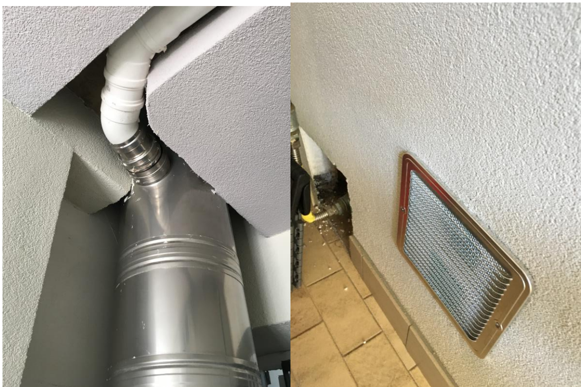
Figure 31. Integrated ducting in the EWI (gas unit exhaust)
