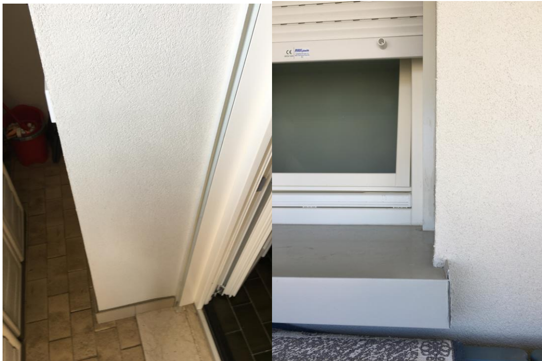
Figure 29. EWI on terraces. Note the reduced space and the toilet window detail.
