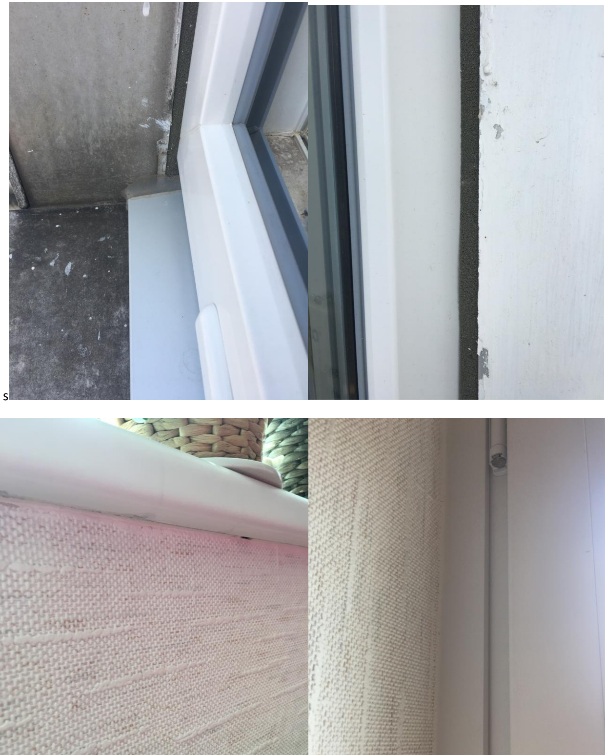
Figure 9. Sealing details on the outside and inside of windows
