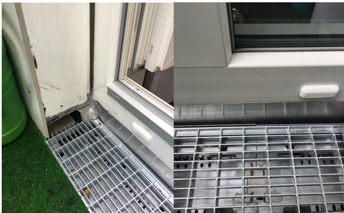
Figure 11. Gutter detail in the door window
