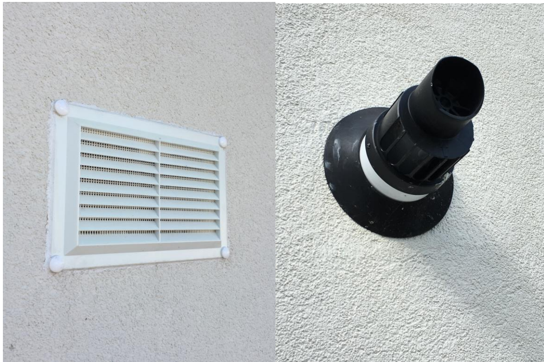
Figure 16. Detail of perforations in the EWI
