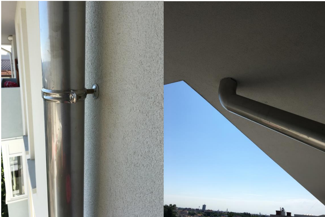
Figure 30. Sealings where the EWI was perforated (fastening and ducting)
