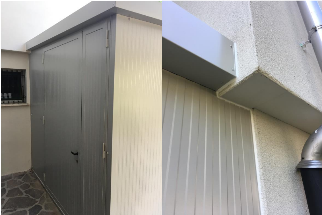
Figure 26. Thermal storage for the solar collectors and joining to the building detail
