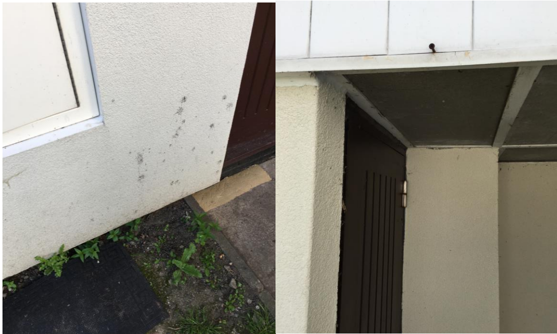
Figure 18. EWI to be washed (left) and part where additional insulation was not installed (right)
