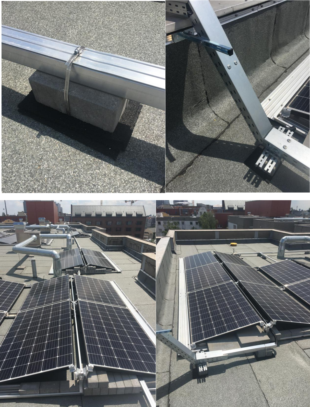
Figure 5. Photovoltaic panels and details of installation structure
