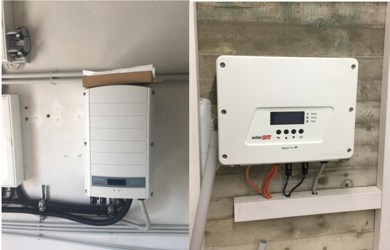
Figure 6. Inverter and batteries for the photovoltaic panels
