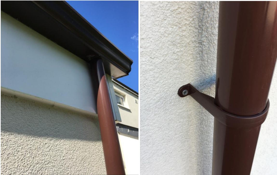
Figure 17. New gutter and fastening detail
