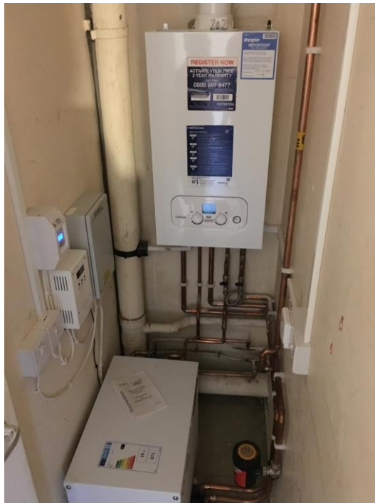
Figure 23. Combination boiler and gel heat storage (the box on the ground)
