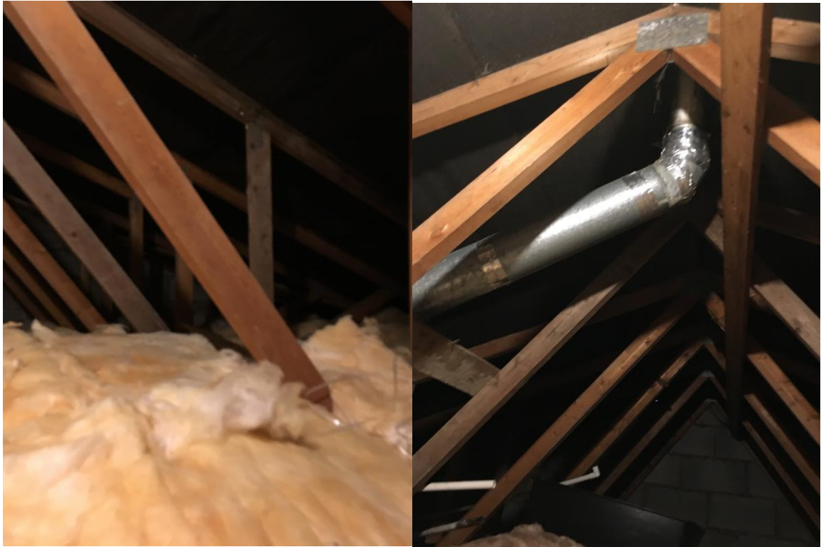
Figure 22. Loose insulation detail (left) and ducting for the gas boiler exhaust (right)
