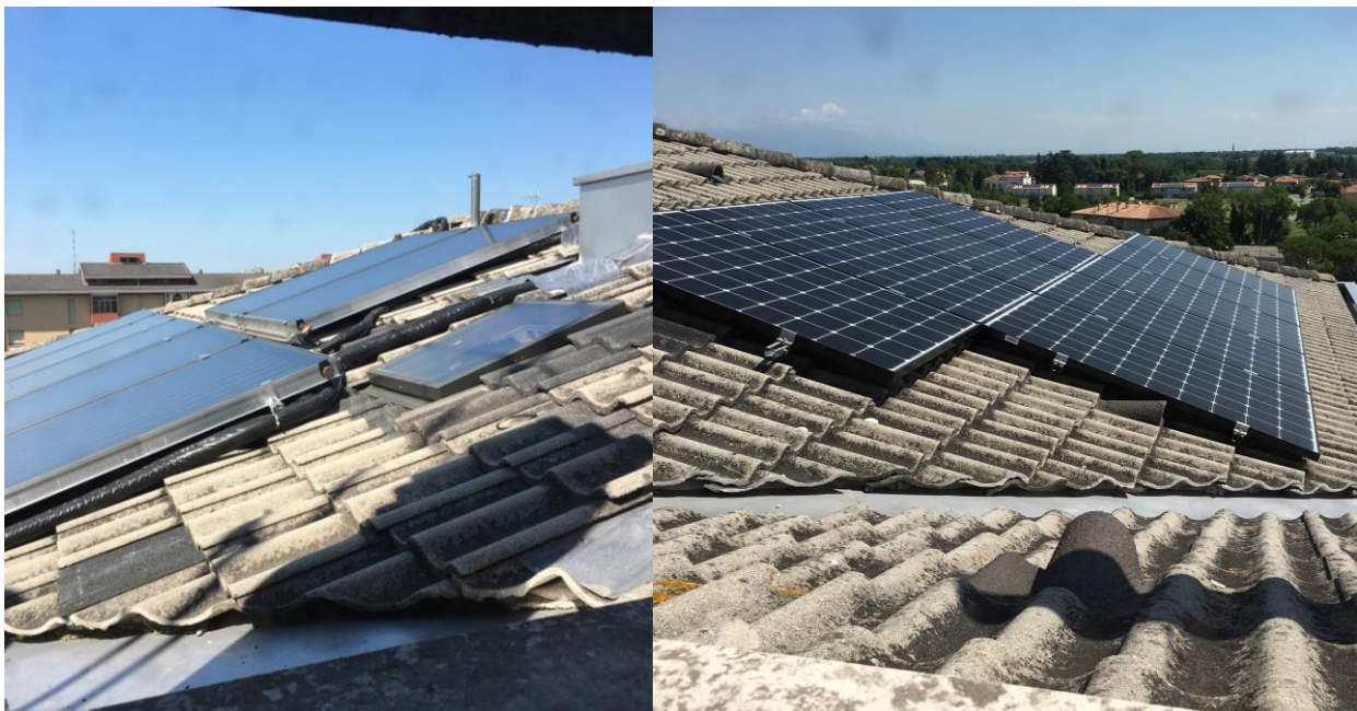
Figure 35. Solar collectors (left) and photovoltaic panels (right)
