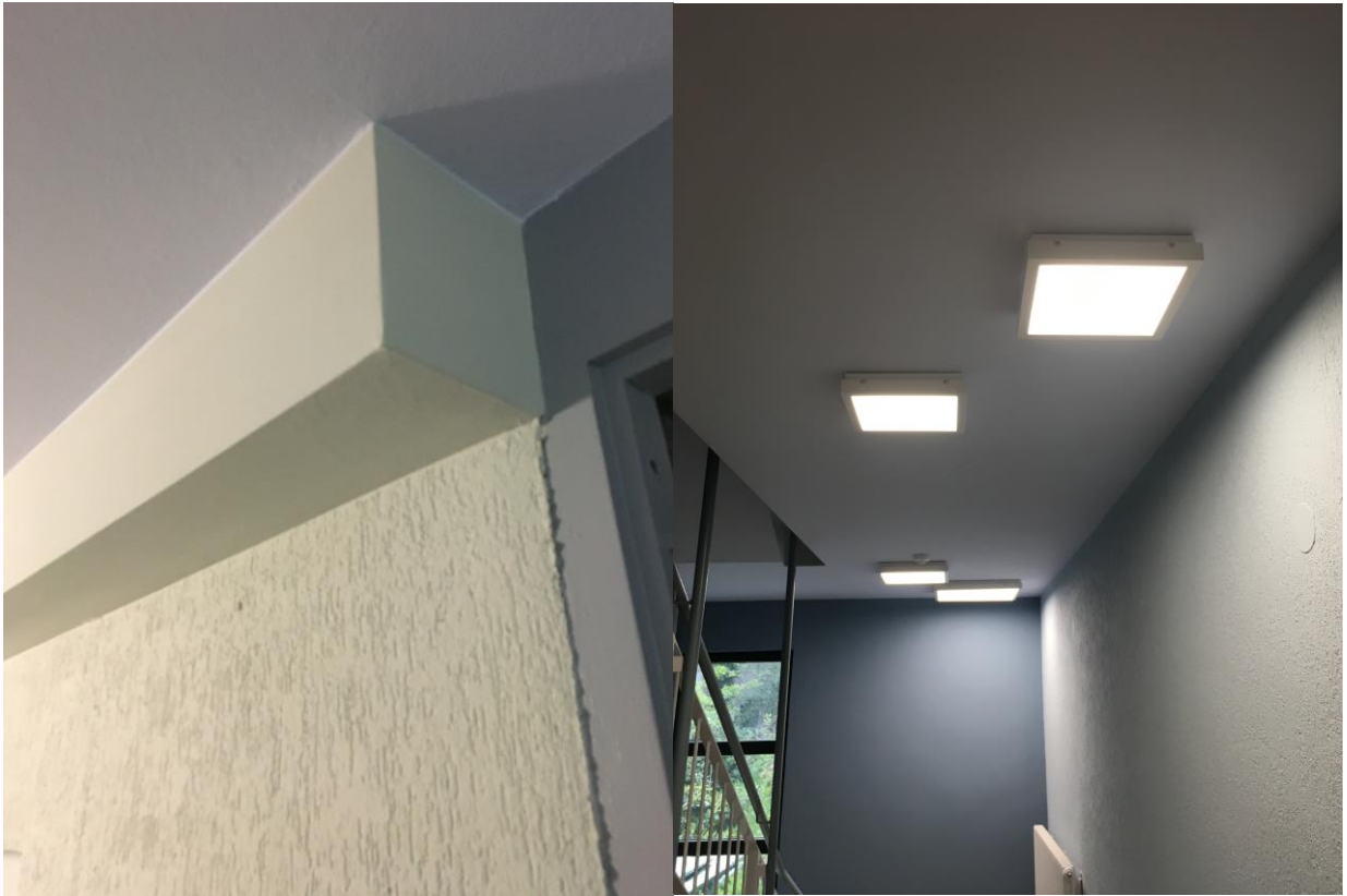
Figure 7. Detail of the cable duct and new led lighting
