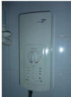
Figure 13: Shower heater thermostat
