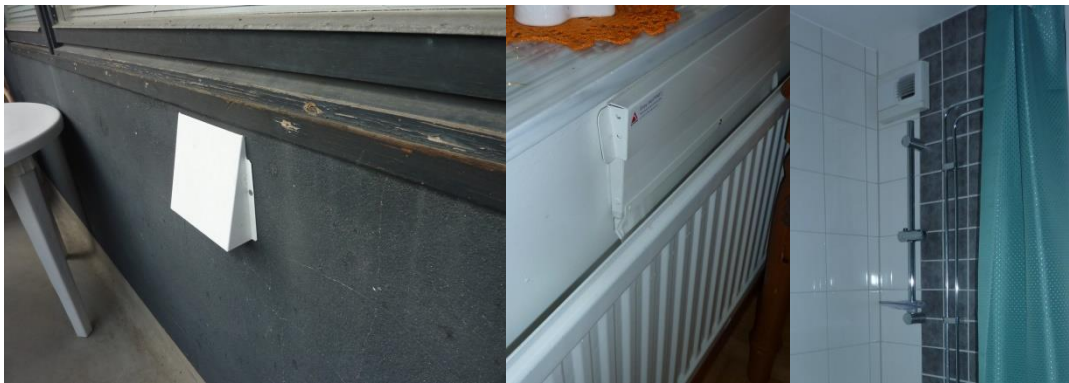
Figure 74: Air Intake/ air outlet in the room and forced ventilation at the rooms
